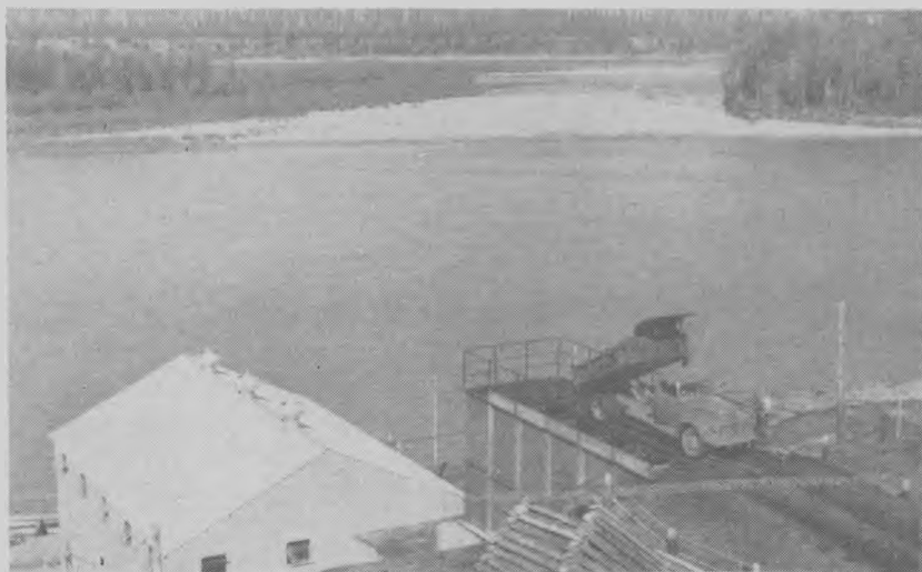
Storage Hopper at Head of Separation Plant
