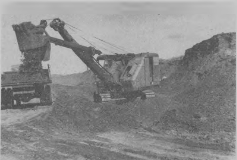
Excavating Oil Sand
