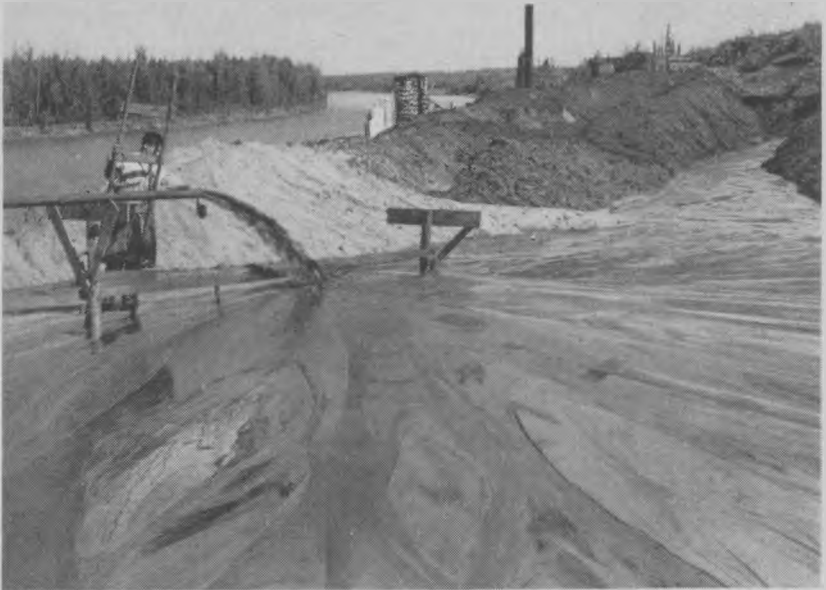
Discharging Sand Tailings to Waste
