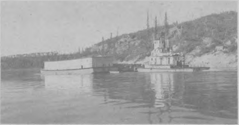
Diesel-Powered Boat and Freight Barges
