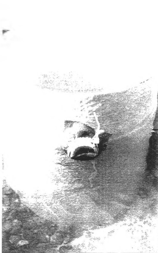
Plate 6. Drain assembly showing (a) fibreglass screen and (b) elbow connection.
