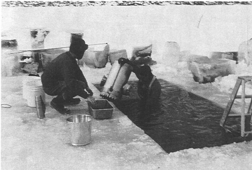
Plate 34. Setting the Neill cylinder without deep water sock. Site 3 - Obed Mountain Coal Bridge.
