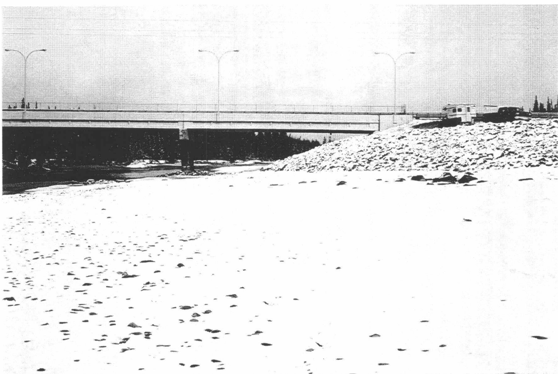
Site 3, near Obed Mountain Road Bridge. Downstream view.
