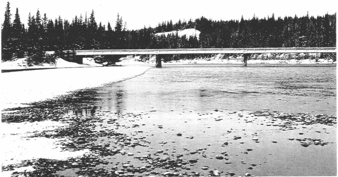
Site 2, near Weldwood Haul Bridge. Upstream view.
